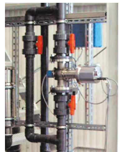
Straight pipe installation with ultrasonic cleaning system
